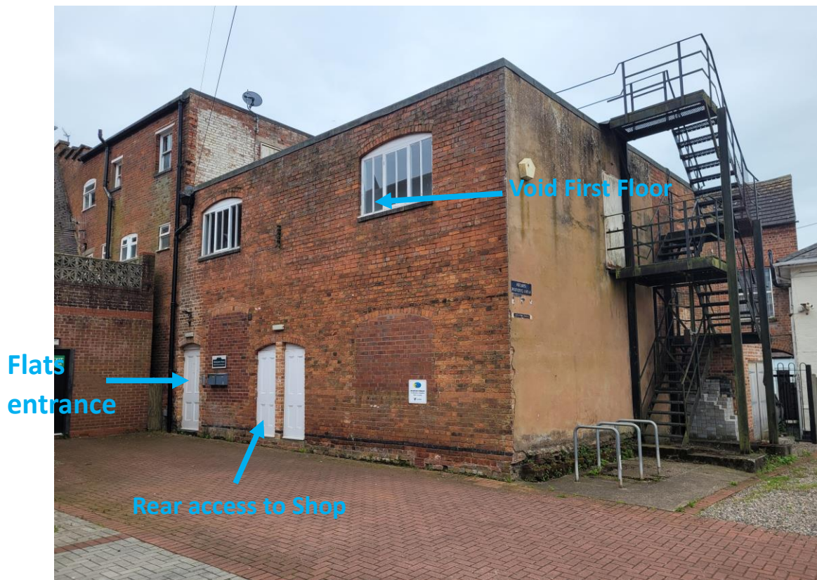
3. Side elevation of rear building having void first floor area
