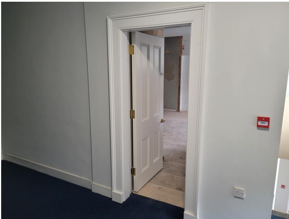
11. Entrance to first floor void area
