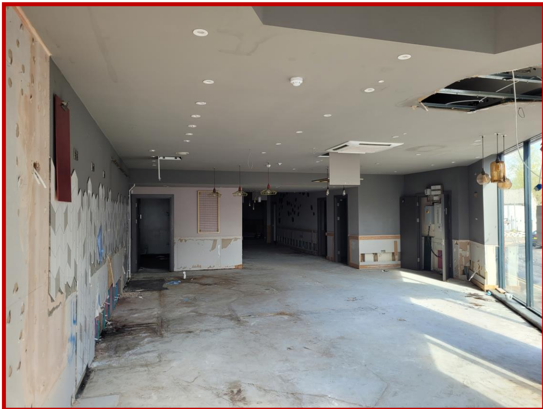
Internal photos of ex Costa – 723a
